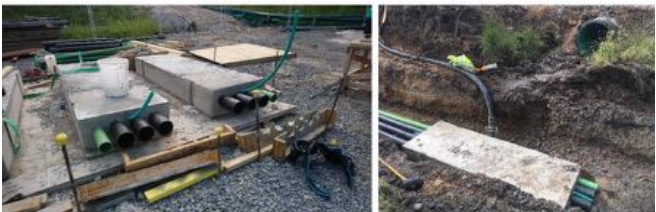
Figure 3 Pre-cast concrete duct blocks manufactured on Morgan Sindall's laydown area (left) and the block in situ being placed underneath a minor watercourse (right)
