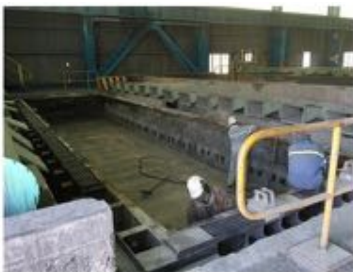
Figure 6: SPL material removed from the cell with sheet metal exposed
